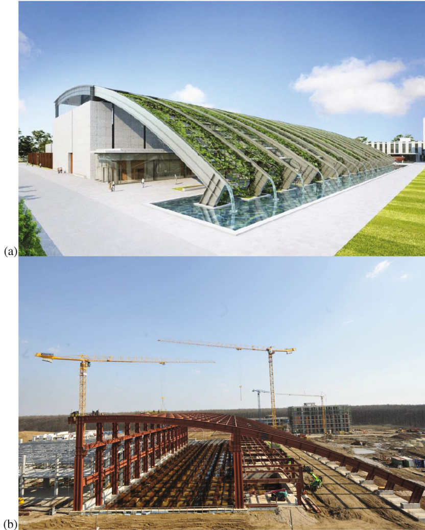
Figure 1. (a) Architect's vision of the main building complex at ELI-NP which hosts the HPLS, GBS and the experiment vaults; (b) status of the construction of the main building complex as on March 2014.
