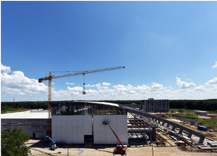
Figure 1: The civil construction stage of ELI-NP in May 2015.
